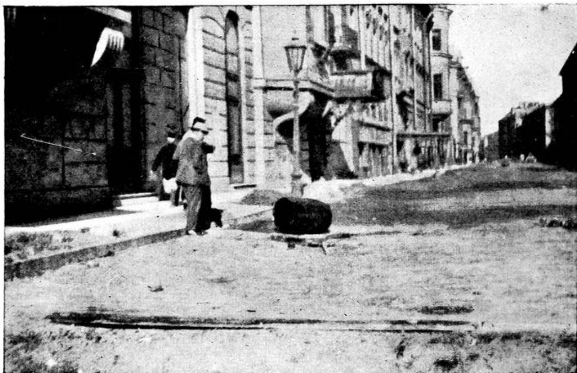
MR. WELLS DISCOVERS A STREET UNDER REPAIR.
